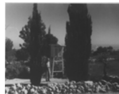
Figure 4b: Har Kenaan station, 1952 looking (photo: IMS archive)
